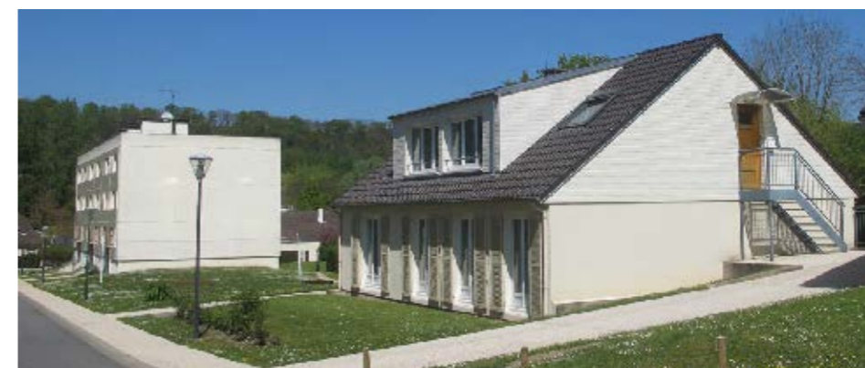
Renovation of one of the pavilion at the Ormaille Residence
